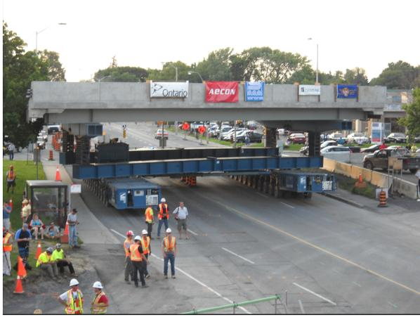
(a) Removing existing bridge decks
