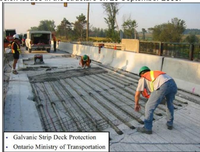
Figure 1: First Trial of DAS Anodes in Bridge Deck Overlay, Ontario, Canada, in 2003
