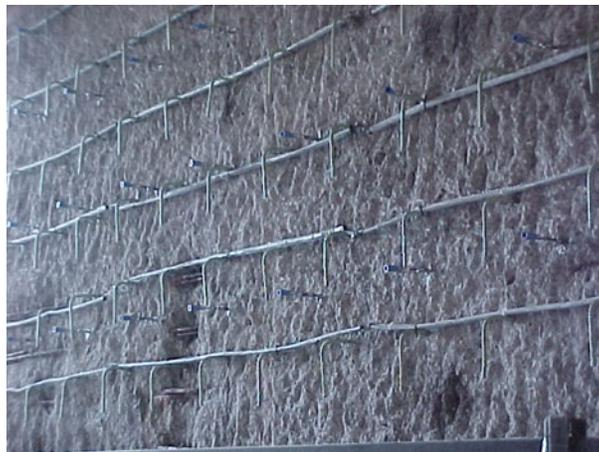
Figure 7 DAS galvanic cathodic protection installation
